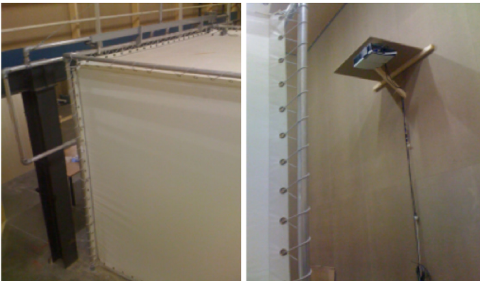
Figure 2; Physical installation of the CryVE system.
